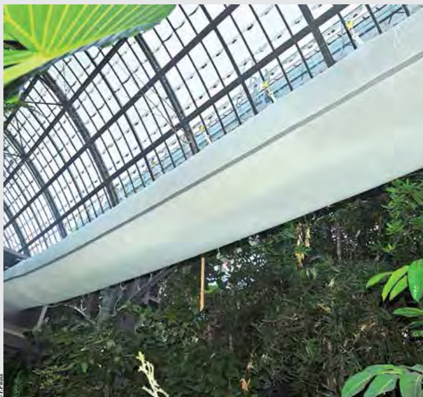
Gaine de chauffage ou "Picoscope"
